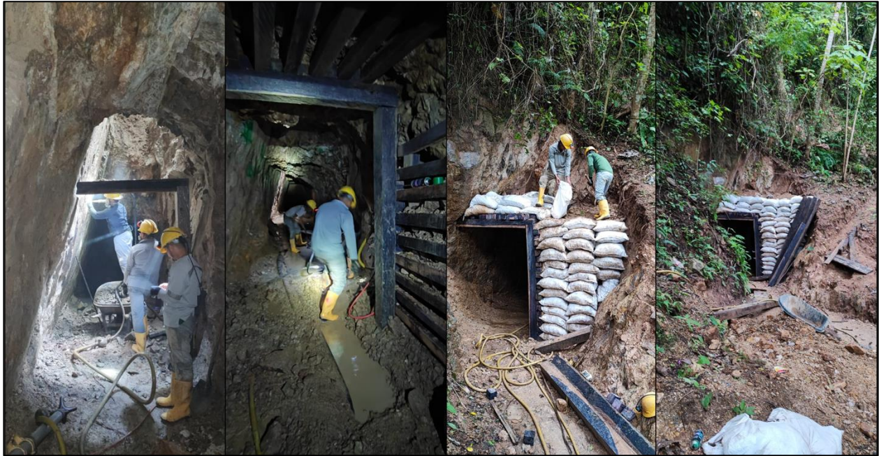
Photo 2. Exploration mine portal and access tunnel rehabilitation at the Mariana Mine.
